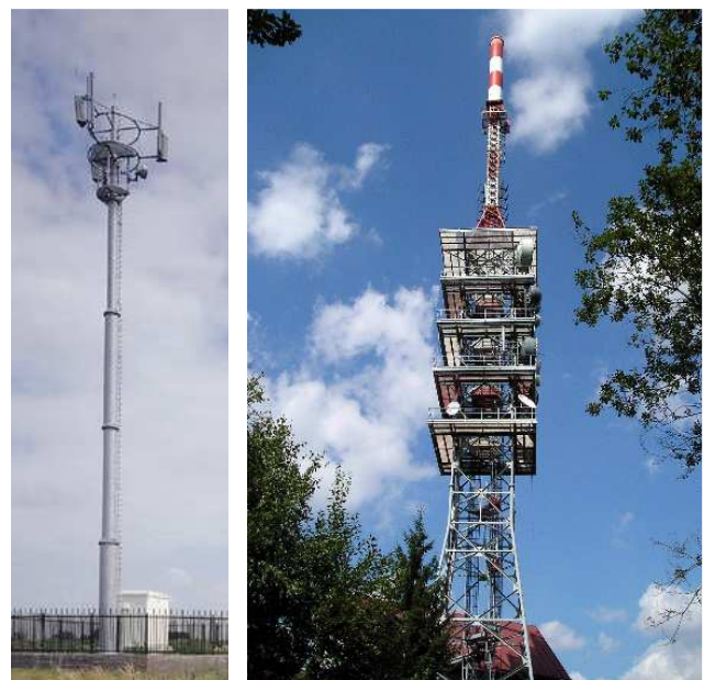
Figure 4: Photo of monopole of height 30 m (left) and of TV tower Vraní vrch with GRP antenna cantilever (right)
