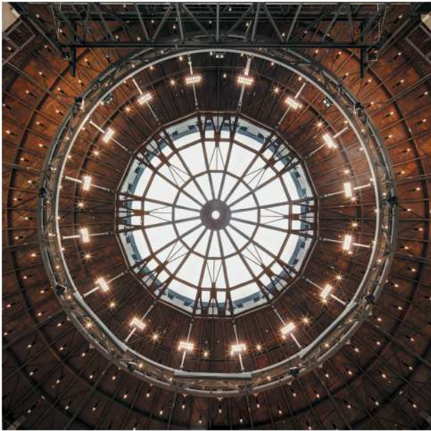
Pohled do klenby, vzpínadlo a otvor ve vrcholu View to the dome, beam string structure and opening in the cap
